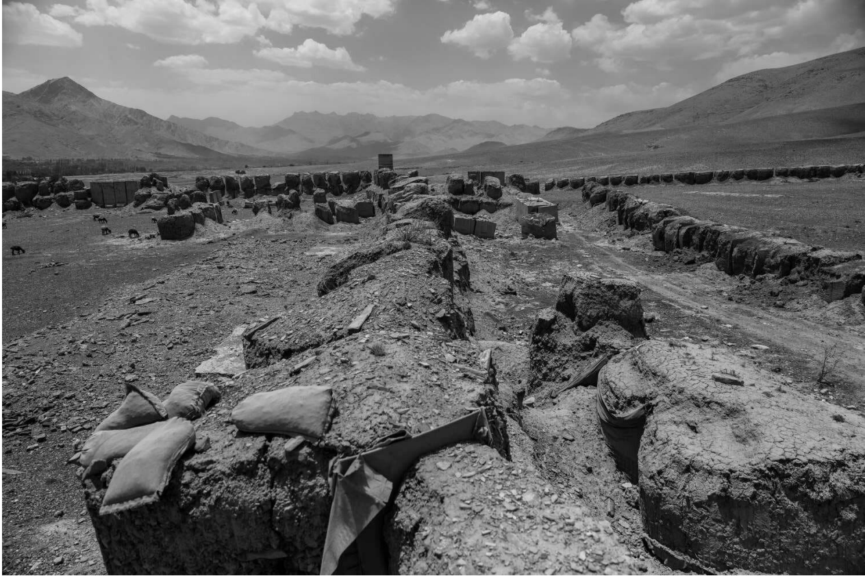
Hesco barriers at an abandoned U.S. Special Forces base in Nerkh in Wardak Province.
